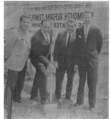
Ground-breaking for the MRT temple building in 1960s.
